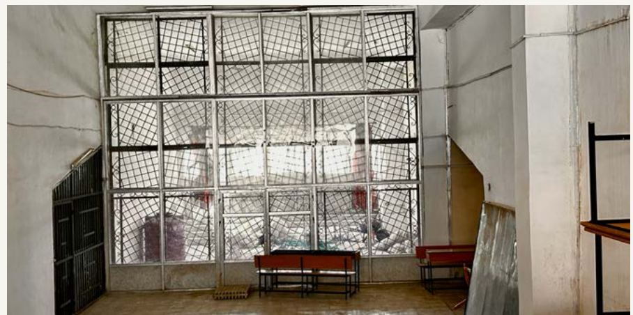
Separated part of a still unfinished building
